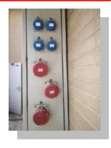
72 fixed 2200W circuits with 16A CEE single-phase outlets, distributed across 4 stage bars, 2 FOH bars, 2 balcony side bars, and 12 floor circuits.
